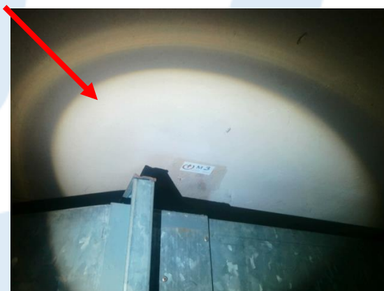
Foto 8 | Brandwerende plafondbeplating
