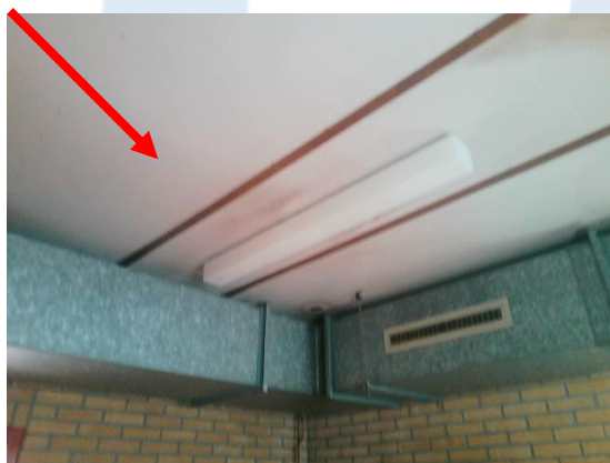
Foto 7 | Brandwerende plafondbeplating
